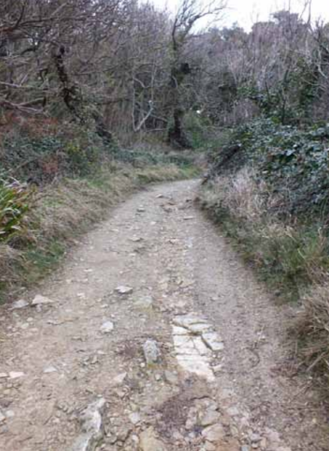
Paths (right) Path surfaces are generally satisfactory but in localised areas such as this, extra drainage needs to be installed to prevent surface water eroding the surface and exposing the rock beneath
